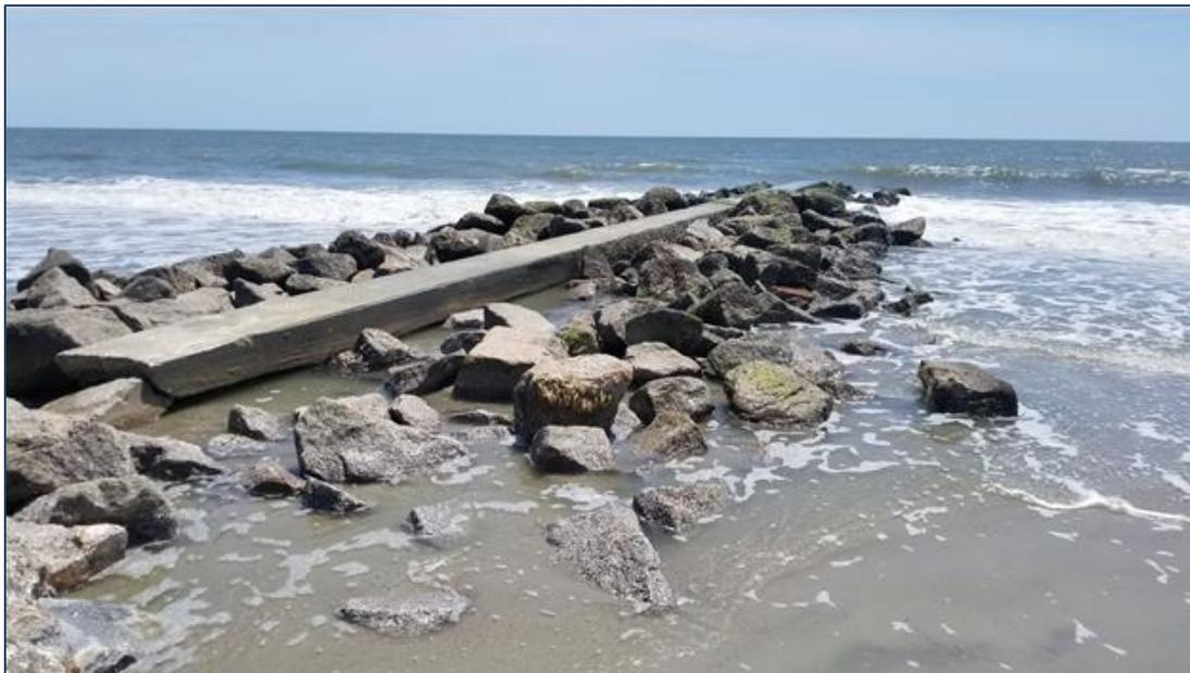
**Figure 1.** Post Irma photos of groin damage. Note the slumped stones below the level of the cap leaving the ends of the structures exposed to wave action.
