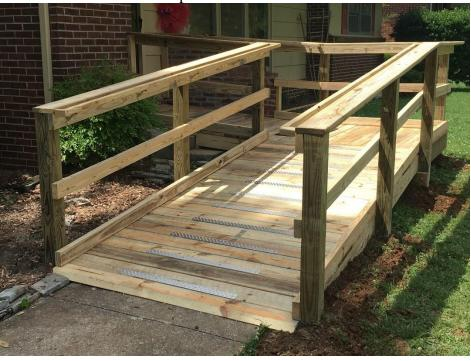
Framing materials were verified on site to be 4x4 posts imbedded in the ground with 2x8 stringers and a 2x6 walking surface. These materials are to be replicated on the newly constructed boardwalks. The approximately 18 feet of curbing should be removed and replicated. All fasteners should be stainless steel. Screws will be used for the walking surface and in any location subject to withdraw.
